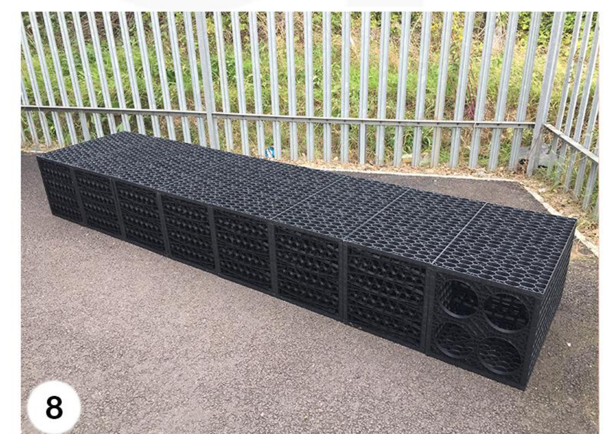
8 Assembly of the crates is now complete.
