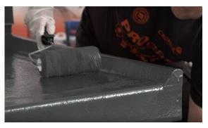
If you are applying a mineral finish, the roof can be left uncoated. Alternatively, you can recoat the roof to create a textured finish. To create a neat finish, mark out any aggregated areas with masking tape, then after the topcoat has fully cured (grabbing the aggregate while doing so), sweep off any excess aggregate.
