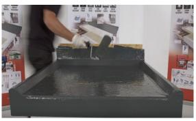
point away from the exit point, using the appropriate sized soft application roller. You should always use latex gloves when handling topcoat or resin.
