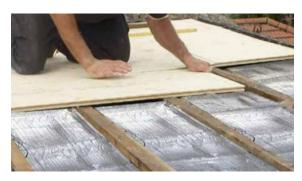
Once the roof has been laminated, the imperfections in the decking will be reflected on the roof surface. You can fix this with gas powered nail gun and 65mm sheradised ring shank nails, alternatively you can opt for a screw gun using plated/passivated woodscrews. Your fixings should be inserted at 200mm spacings on every joist.
